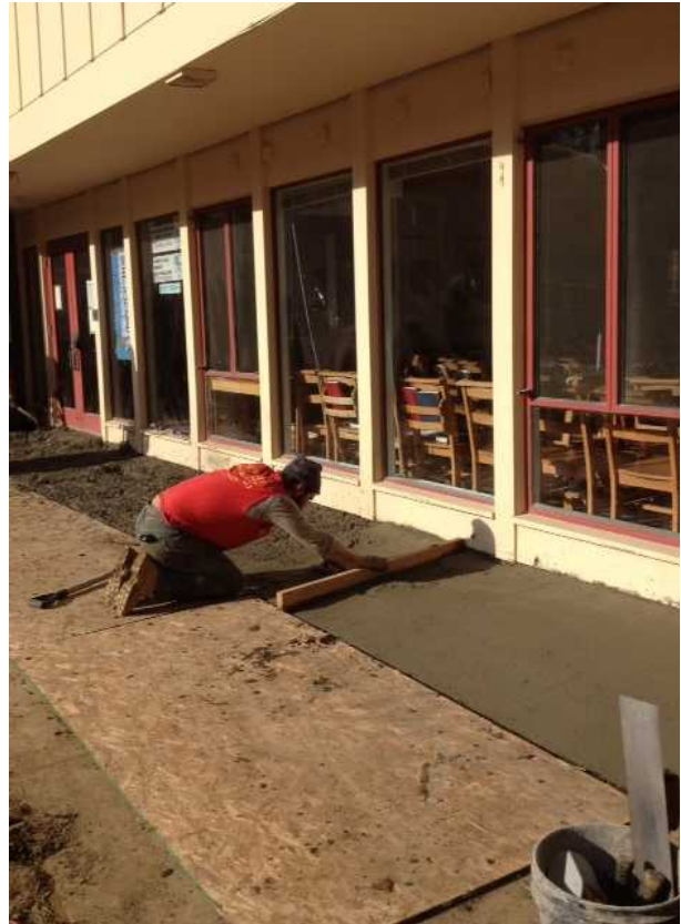
The new walks being finished.
