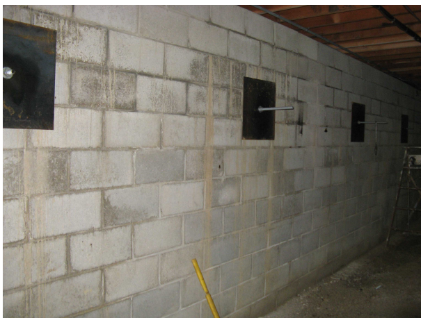
The basement wall, not going anywhere
