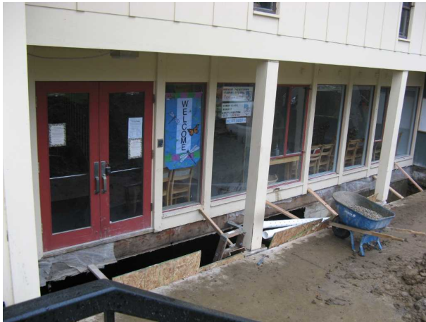
The new walks excavated
